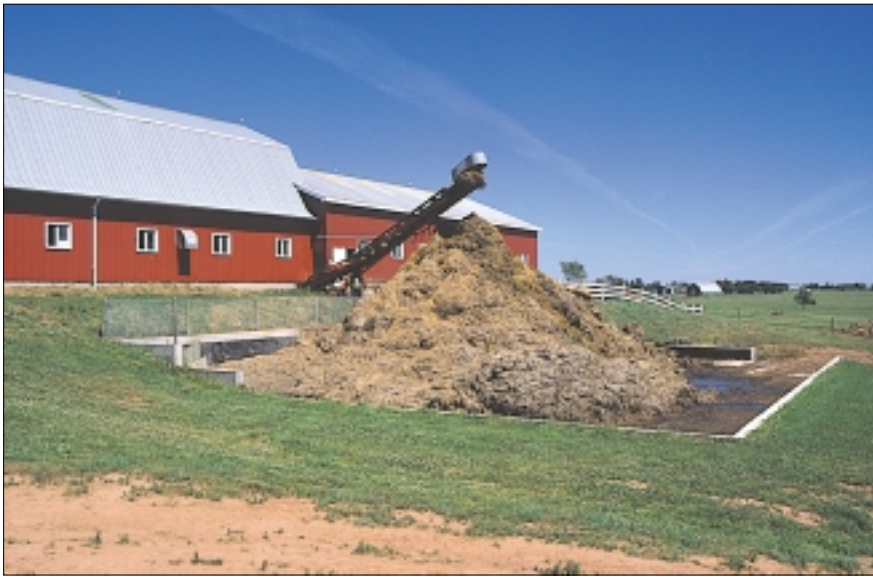
Solid manure storage - curbed concrete slab with ramp.
