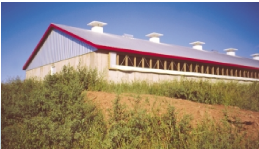
Roof exhaust outlets to maximize air dilution.
