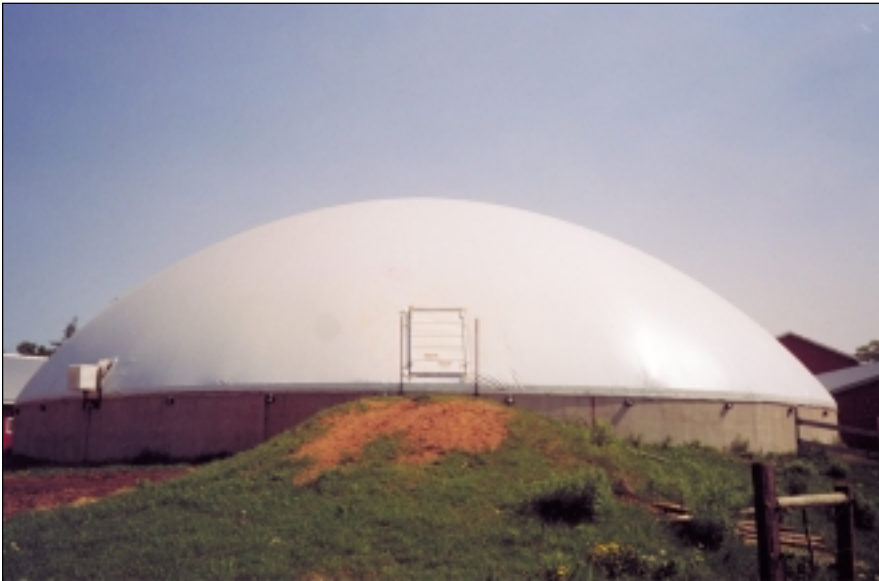
Concrete liquid manure storage, with cover for odour control.
