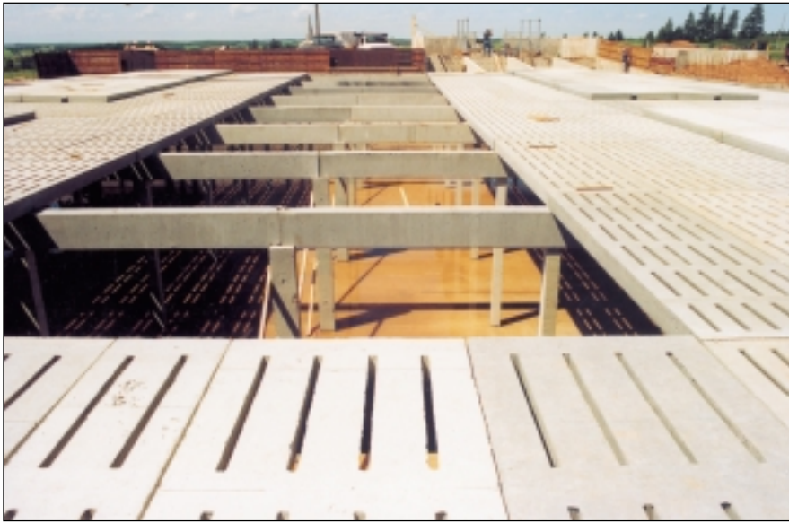
Liquid manure storage - underbarn concrete storage with slatted floor (under construction).
