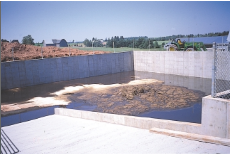
Curbed concrete manure storage with safety fence.
