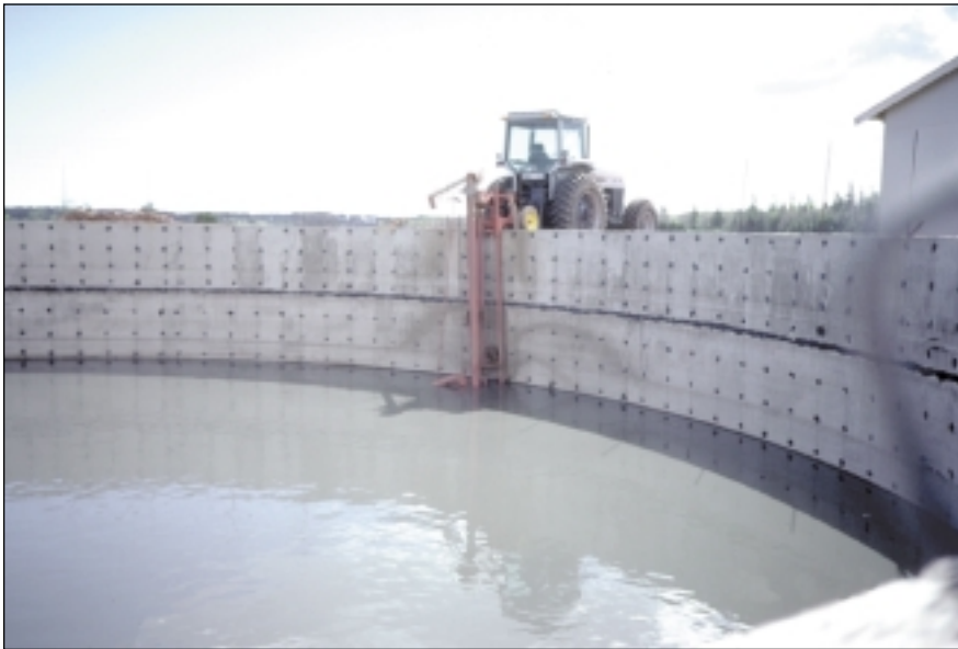
Liquid manure storage - circular concrete tank.
