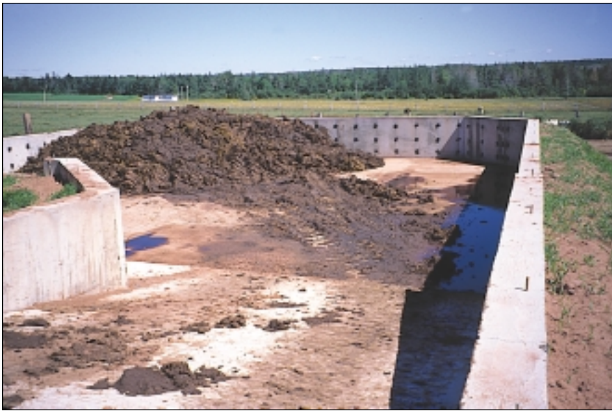
Solid or semi-solid manure storage - concrete slab with sidewalls and drive-in ramp.
